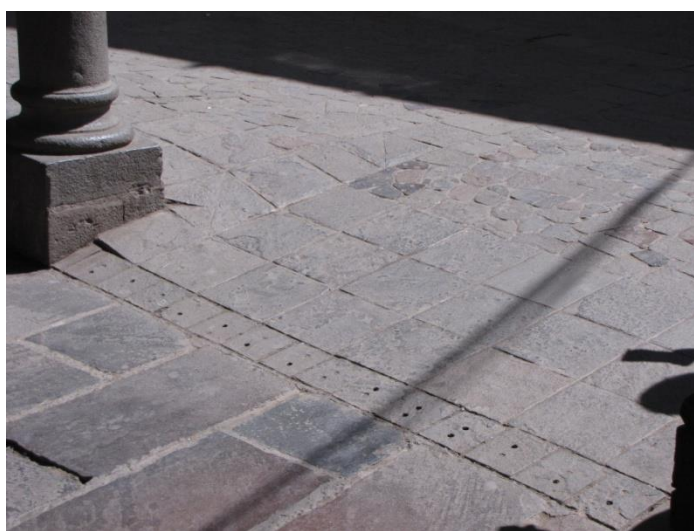
PORTAL COMERCIO, RAMPA PEATONAL
