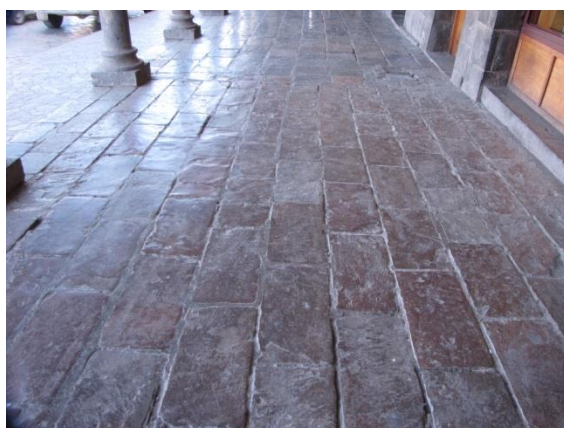
PORTAL DE PANES, LOSETA REGULAR RECTANGULAR TRASLAPADA
