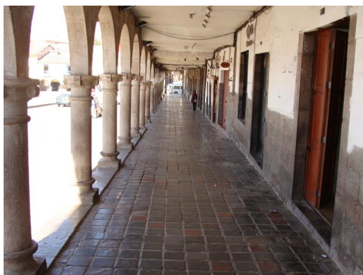
Vista general Portal Panes
